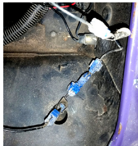
Four splices in just one short section of taillight wire.
