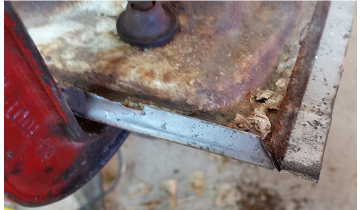
The bottom edge of the patch already had the folded edge. After 45 degree relief cut is made. The forming process is continued on the second edge.
