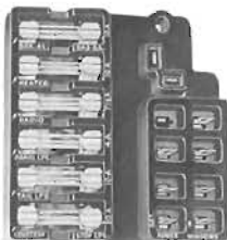
Typical Fuse Block
