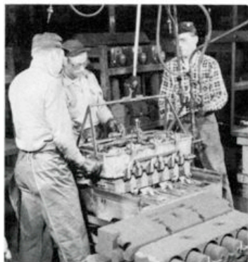
Removing cylinder block casting from sand mold.
