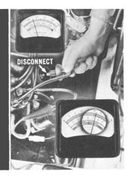
If the customer has made a serious complaint about excessive fuel consumption, it is suggested that the vehicle be road-tested with a Gas-per-Mile Gauge such as J-8381. Specific instructions are packaged with the unit and are also described in detail in the Chevrolet Service News of November, 1959, Pages 4 and 5. The mileage test should be made with the customer present and will help show any unusual driving habits which have contributed to the poor mileage complaint.
