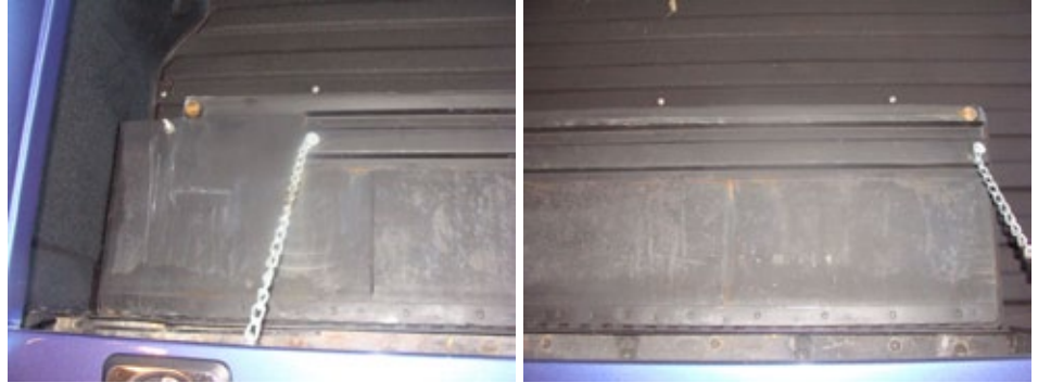
You can see in the left hand picture, the welded joint just right of the body line. The notch at the top left is to clear the cab overhang.
