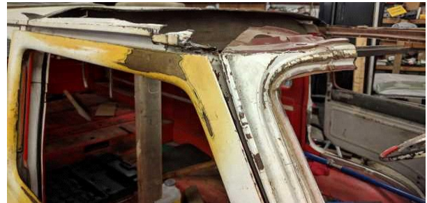
Pass. side front with alignment references and identified issues.
