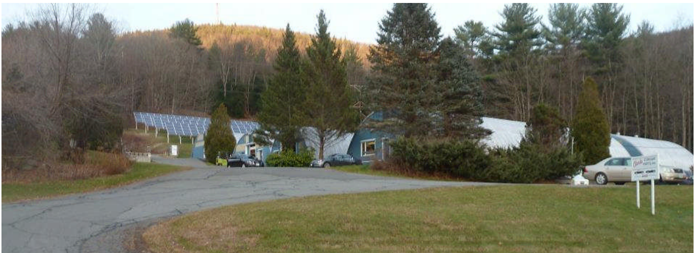
Photo by Jonathan Rintels: Here is a photo of the Clark’s Corvair facilities in Shelburne Falls, Massachusetts. In December 2012, Jonathan wrote, “Cal has installed new solar panels that when the switch is thrown should provide more than enough power for his entire operation – and more! The cutting edge of modern tech – solar energy – meets the cutting edge (well, sort of, kinda) of 1960 s auto technology, the Corvair.
