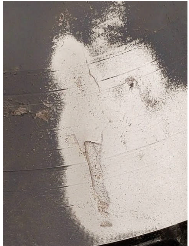
Sometimes, you'll see cracks and corrosion on the bottom side of the fan, too.
