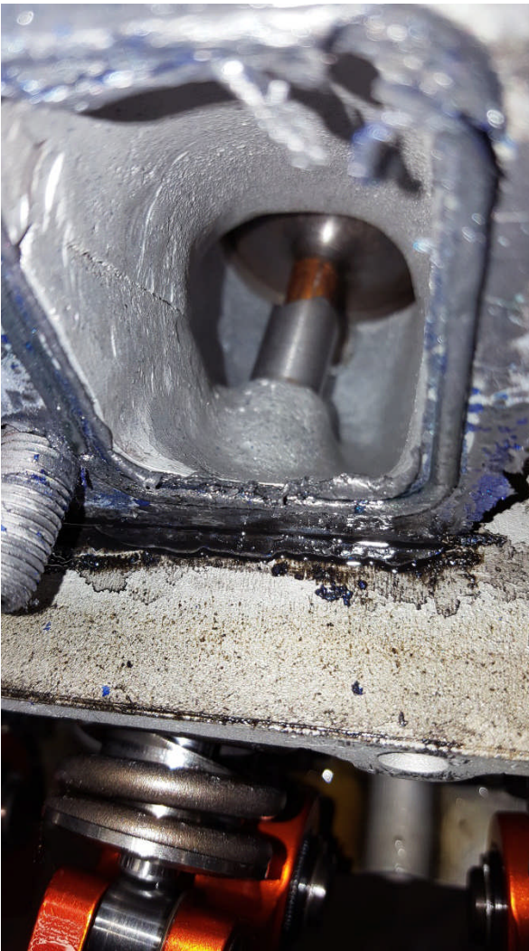
Left Photo: BROKEN GUIDE
