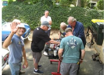
Before the 140 engine was brought outside, Bryan, with his converted-to-a-tool distributor shaft, used it with a drill to build up oil pressure while Byron turned the crank over one rotation so all journals got hit with oil. With one more rotation, it was back to #1 cylinder at TDC so the distributor went in with Jimmy's borrowed Point's Plate.
