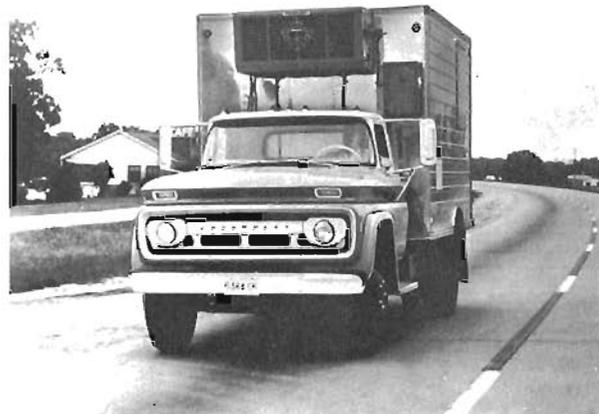
Radiator shutters are available as an option for D60 models this year.\* They keep engine temperatures in the most efficient range under a wide variety of operating conditions.
