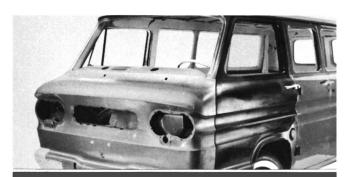
The straightened and rewelded body shell is now ready for painting. The front suspension, gasoline tank and steering gear assembly have been installed. Other parts will be connected and attached after painting. This completes Major Front End Damage Repairs.
