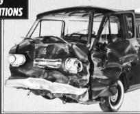
Serious damage is indicated on the lower underbody structure, on the interior, and —
