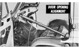
The left front cowl pillar was pushed forward at the belt line, using the diagonal jack setup shown. This restored door alianment.
