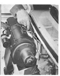
Before disassembling or removing any parts from a burner, note the condition or appearance of the mixer cup, which is very often a clue to the cause of unsatisfactory operation. In a properly operating burner, the end of the nozzle around the orifice will be gray—the inside of the mixer cup around the nozzle will be covered with a medium layer of carbon. The outer end will be burned to a gray or reddish color, and some scaling of the mixer cup will have taken place.
