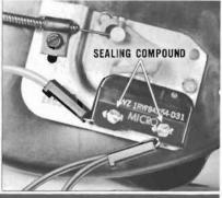
heater output or a burned out heat exchanger. The factory adjusting screws are sealed with compound to prevent changing the adjustment.
