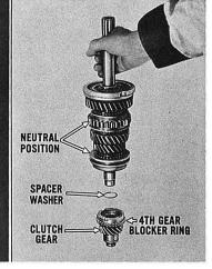
Clamp the mainshaft in a vise with the forward end of the shaft upwards. Remove the special snap ring, the 3-4 synchronizer and 3rd gear blocker ring from the shaft. Remove the 3rdspeed gear, the needle-bearing thrust washer, the 2nd-speed gear, and the 2nd gear blocker ring. SNAP RING 3-4 SYNCHRONIZER 3RD GEAR BLOCKER RING 3RD GEAR 9RD GEAR 0 NEEDLE-BEARING THRUST WASHER 2ND GEAR LOCKER RING
