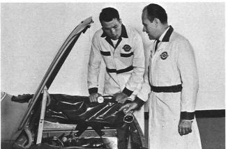
Block the choke and throttle valves wide open; then I'll crank the engine over for you. If you find compression weak in any cylinder, there's no point in going any further with the tune-up. O.K.?
