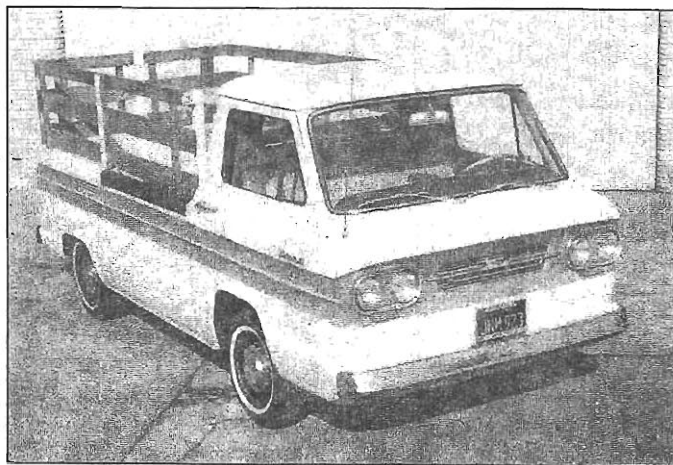
Corvair vans and pickups used a "forward control" design that allowed the driver to sit above the front wheels, since the engine was placed in the rear. Note the rampside door on the passenger side of this 1961 model. (David Gooley photo)
