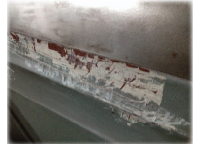
Over the years seven layers of paint had been applied and porthole windows installed. The windows stay but the paint is coming off.
