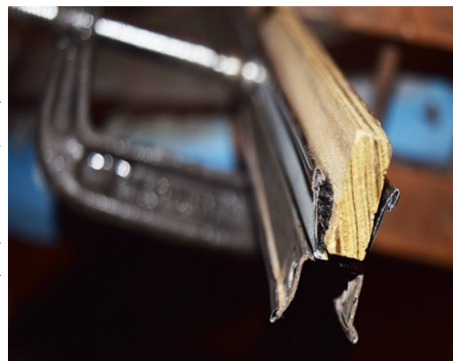
Figure 3. Backer wood strip in channel.
